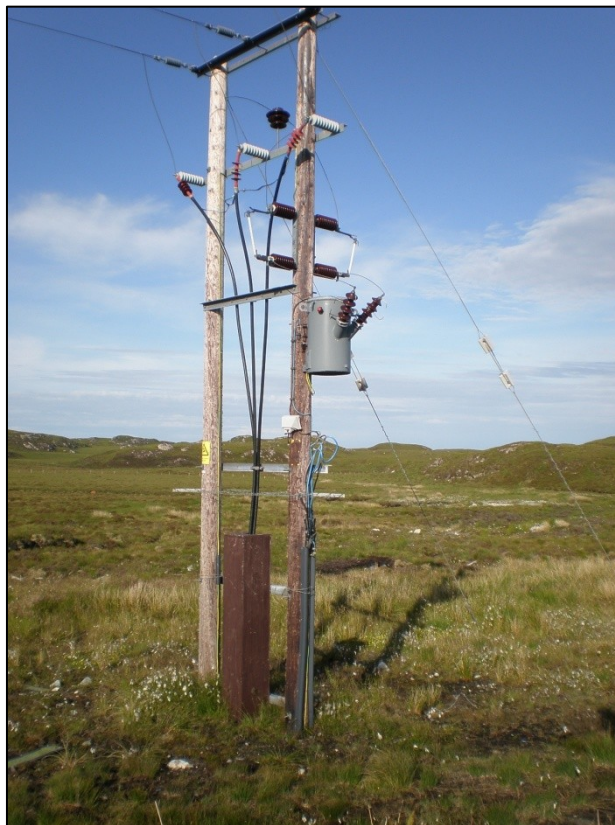
Figure 2-2: An example of a 33kV wood pole structure with cable terminations and 33kV to LV pole mounted transformer
