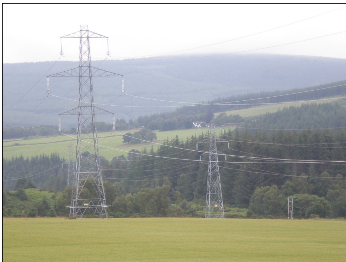
Figure 2-1: Example of a 275kV, a 132kV and 33kV line (left to right)
